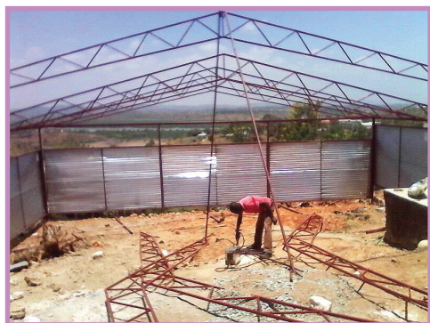
New home of Mombasa Grace School of Ministries under construction
